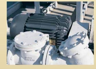
A Totally Enclosed Fan-Cooled (TEFC) motor refers to an industrial electric motor equipped with an external fan to circulate outside air to the motor. A TEFC motor offers increased protection against weather, dirt and moisture that will help prevent motor failure and extend motor life.
